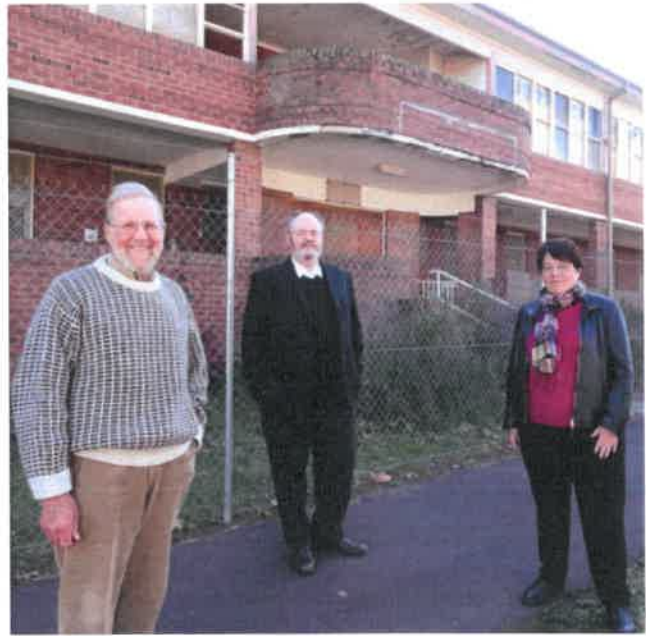
Historical Society members Euan Greer and Liz Edwards with James Nicholson of Adaptive Architects Pty Ltd outside the former nurses' quarters in Sale Street.
