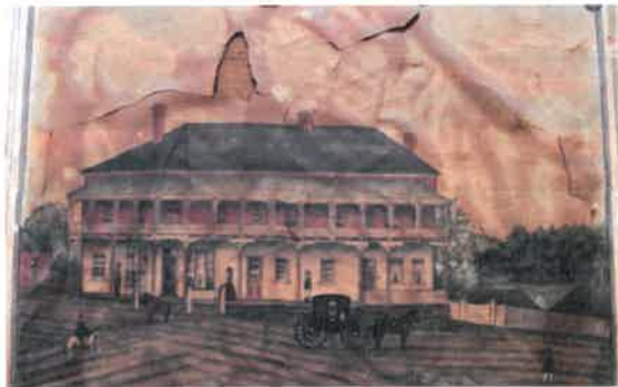
Hirst's painting is in perilous condition but clearly shows the building as it was in 1872.
