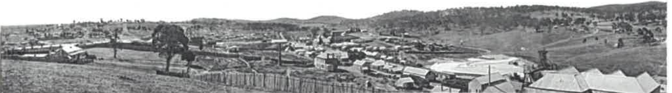
The first of two Lucknow panels.
