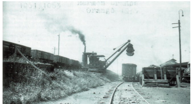
Image 4. The old depot at the station in 1933. Steam coal grabs are coaling the tender of a locomotive from the trucks on the track behind. The engine shed roof is seen in the right background. SRA Archives from Love (1998), p.9
